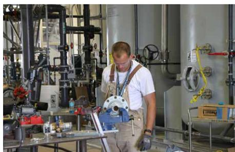
A pipefitter in the 200 West Pump and Treat's Radiological Building is installing a uranium treatment system, which consists of a series of ion exchange columns.
