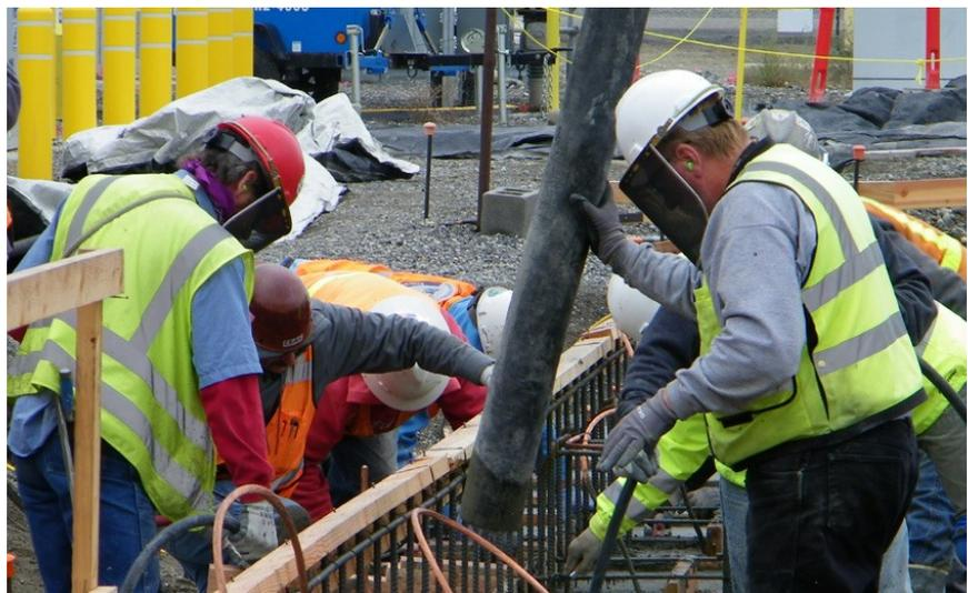
Concrete placement for the K West Annex building that will house the sludge retrieval equipment.
