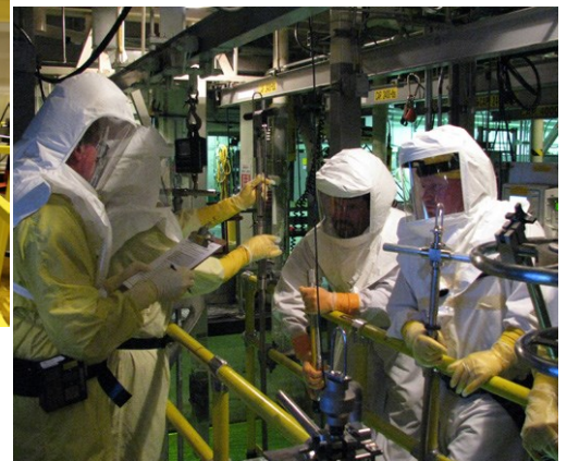
(Left) At MASF, workers practice with long-reach tools that will be used to retrieve sludge from the K West Basin. (Right) Workers deploy sludge retrieval tools at the actual reactor.
