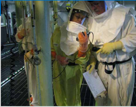
Workers in safety gear prepare the basin to receive sludge removal equipment.
