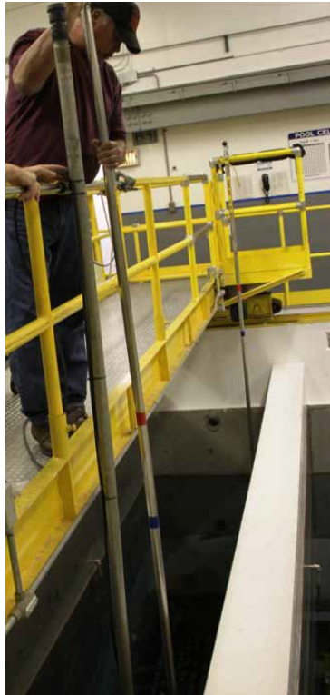
Workers used long-reach tools (left) and video technology (right) as they repositioned the capsules to reduce the heat load of the capsules in underwater storage at WESF.
