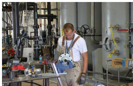
A pipefitter in the 200 West Pump and Treat's Radiological Building installs components to remove uranium from groundwater.
