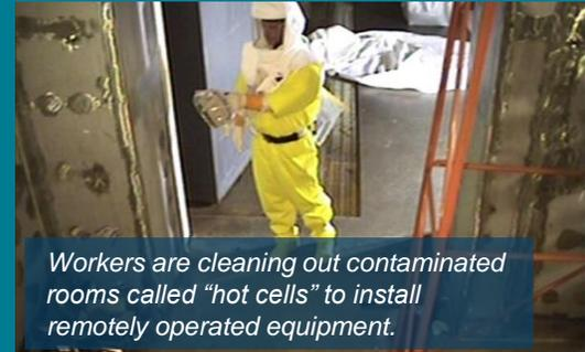
Contamination is estimated to extend 6 to 8 feet below the B Cell floor. Radiation levels are so high that remotely operated tools must be used.
