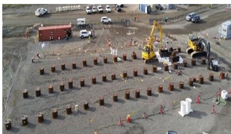
For 80 of the 94 vertical pipes, workers drove overcasings around the pipes, and an auger removed the pipe, the contents inside, and the soil inside the overcasing.
