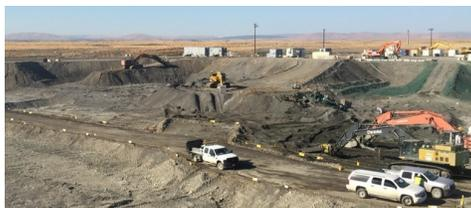
Excavators removed soil to expose vertical pipe units (VPUs) filled with waste.
