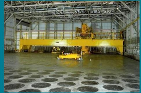
*A crane inside the 42,000-square-foot CSB is used to lift multi-canister overpacks from belowgrade concrete vaults.*
