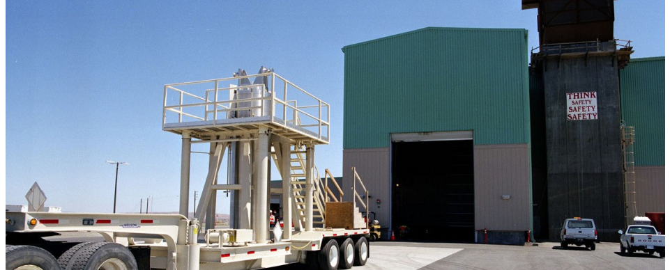
Delivery of high level material to the Canister Storage Building.
