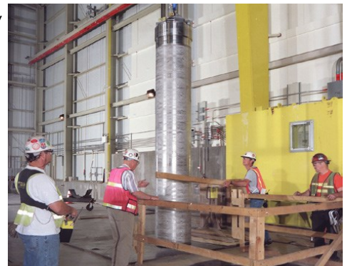
Workers handle an empty multi-canister overpack.
