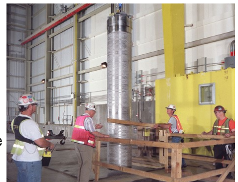
Workers handle an empty container, called a multi-canister overpack, used to store irradiated reactor fuel.
