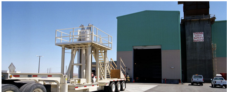
High-level radioactive material is delivered to the Canister Storage Building.
