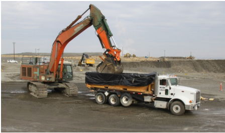
Containers are filled with waste to be disposed of at ERDF.
