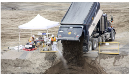
Workers safely dispose of waste at ERDF.
