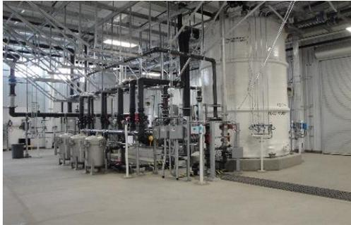
*Ion exchange treatment train removes uranium and technetium-99 from the groundwater at the 200 West Area Pump-and-Treat Facility.*
