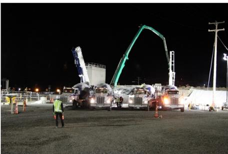
On Oct. 1, 2017, workers began placing engineered grout inside PUREX Tunnel 1 to stabilize the partially collapsed tunnel.
