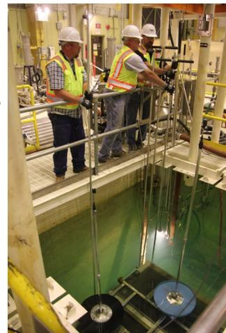
At a replica facility, workers train with tools and techniques that will be used to retrieve highly radioactive sludge.
