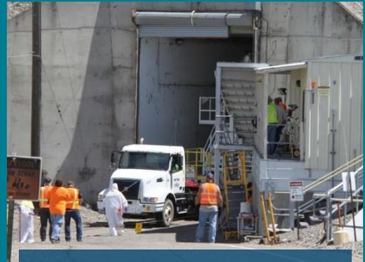
*A truck and trailer hauled sludge containers from the 100 K Reactor Area to T Plant for storage.*
