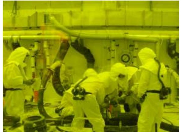
Workers recently stabilized legacy contamination inside WESF, an early step in preparing the facility to transfer the capsules to dry storage.
