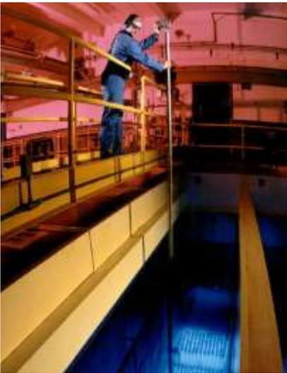
The water around the cesium and strontium capsules in the Waste Encapsulation and Storage Facility pools glows a color of blue. The effect is known as the Cherenkov Glow, as the radioactive cesium and strontium decay and lose their radioactivity to become stable atoms.
