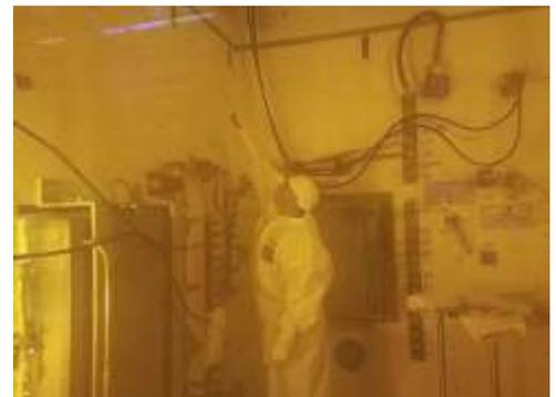
Workers recently decontaminated and painted a hot cell adjacent to the WESF pool cells where the capsules will be transported to a safer storage configuration.
